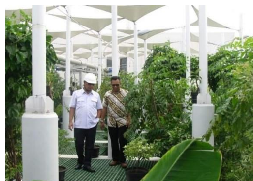
Figure 1. Canopy steel and trees on the wastewater treatment
