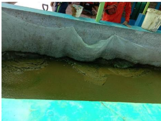
Gambar 5: Sludge Drying Bed
